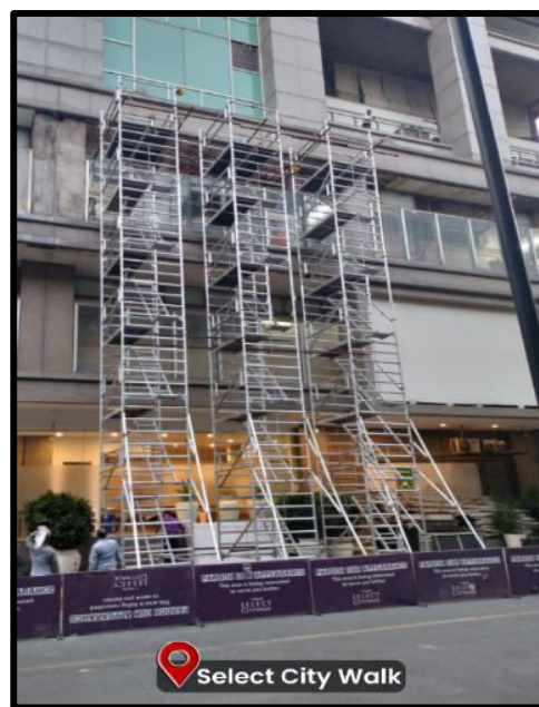
Rental supply of Aluminium Scaffolding (Model MST125-06 and 2.5m Bridge Sections) at Select City Walk Mall, Saket, New Delhi
